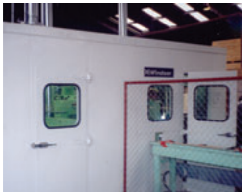
Acoustic enclosure in sawmill
