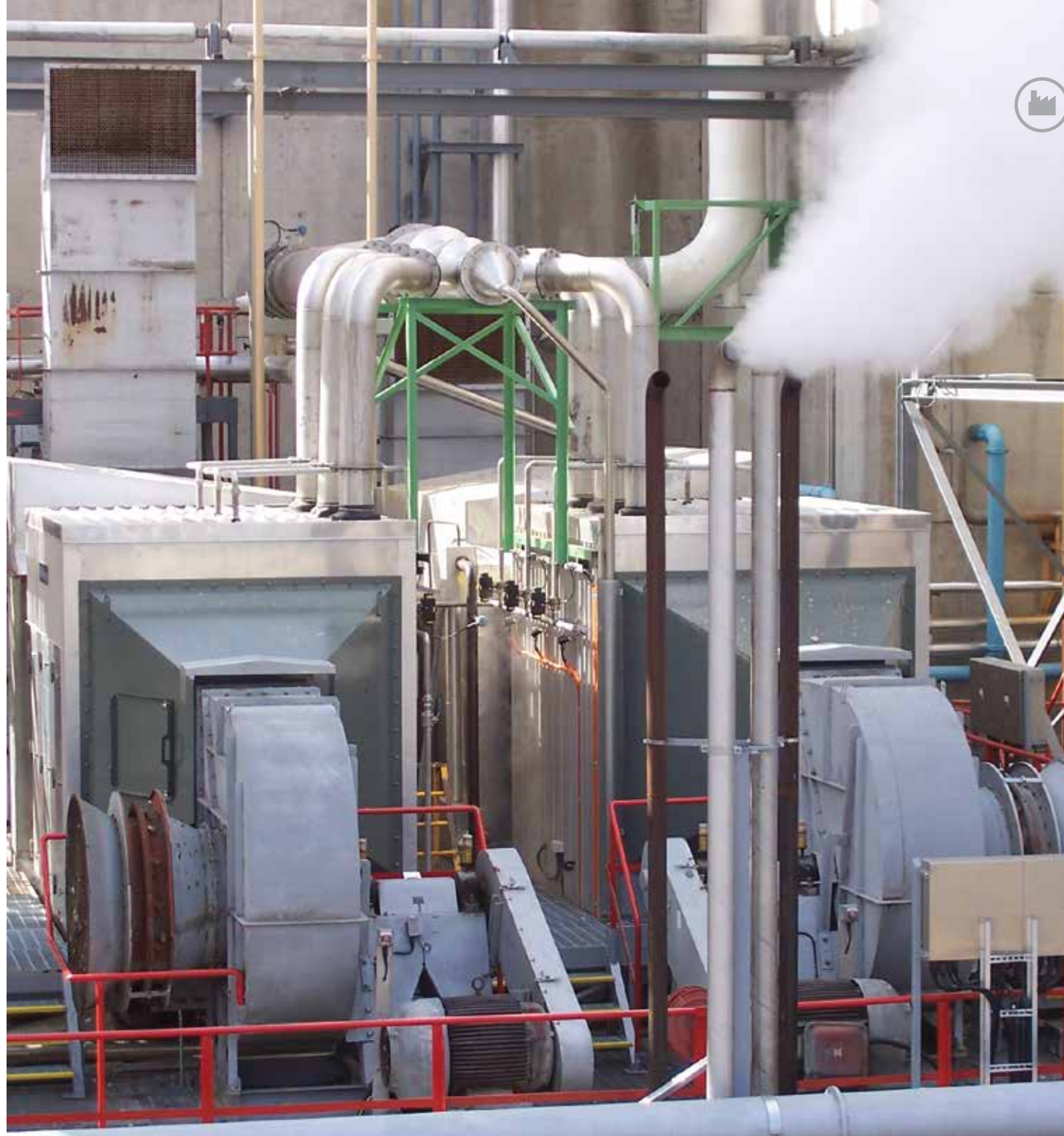
Two Windsor waste steam recovery units at a pulp mill in New Zealand.
