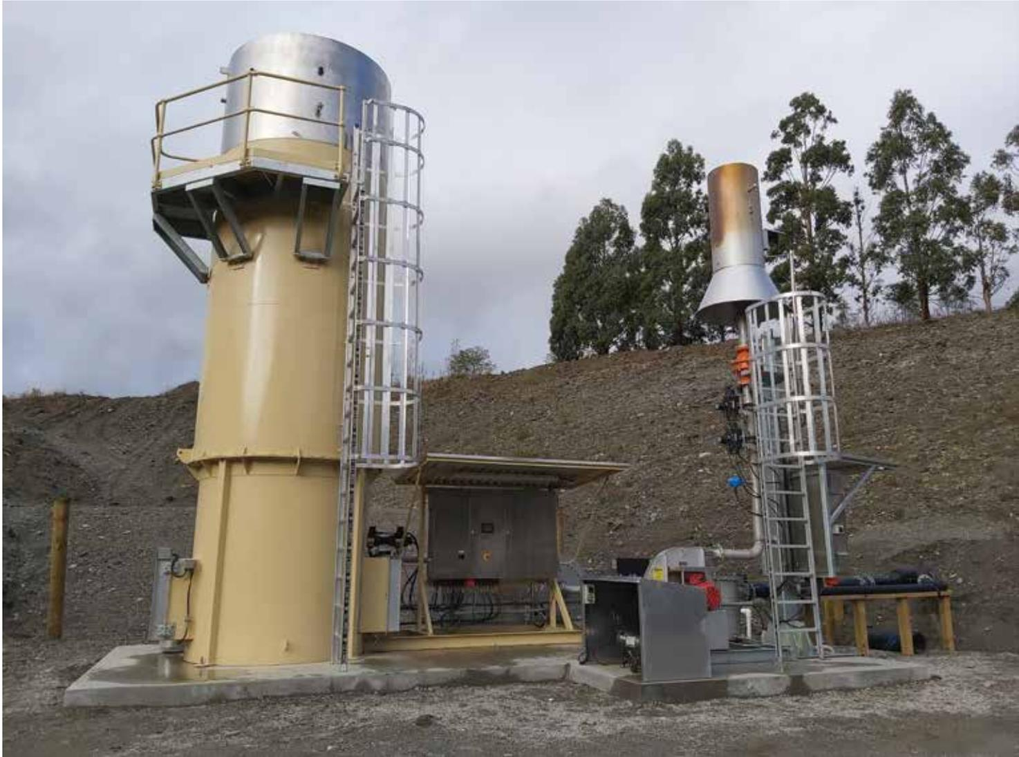
Utilising waste gas in process heating or power generation (gas engine) is a preferred method of disposal, but it is sometimes impractical due to distance from a suitable site. Gas may also need a secondary method (stand by) of disposal or the need to be load balanced with other equipment. Burning gas in a Windsor gas flare can be an excellent option in these situations.
